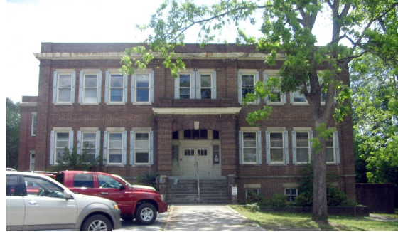
Front elevation of the Oconee Street School
